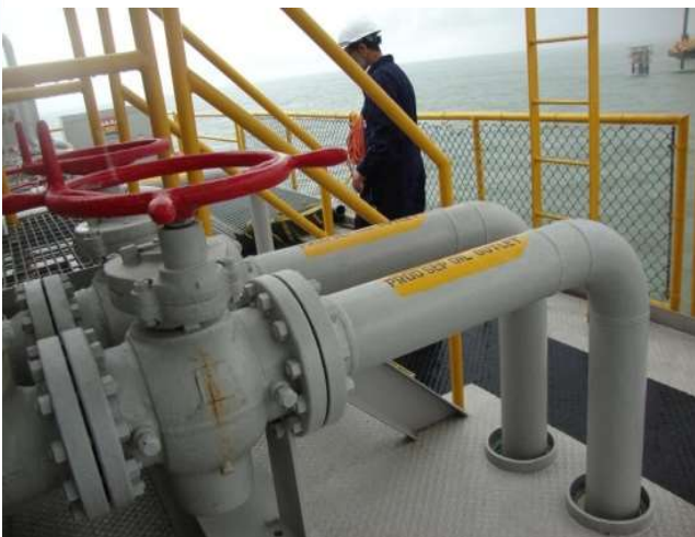
Installation Work executed by BGV
