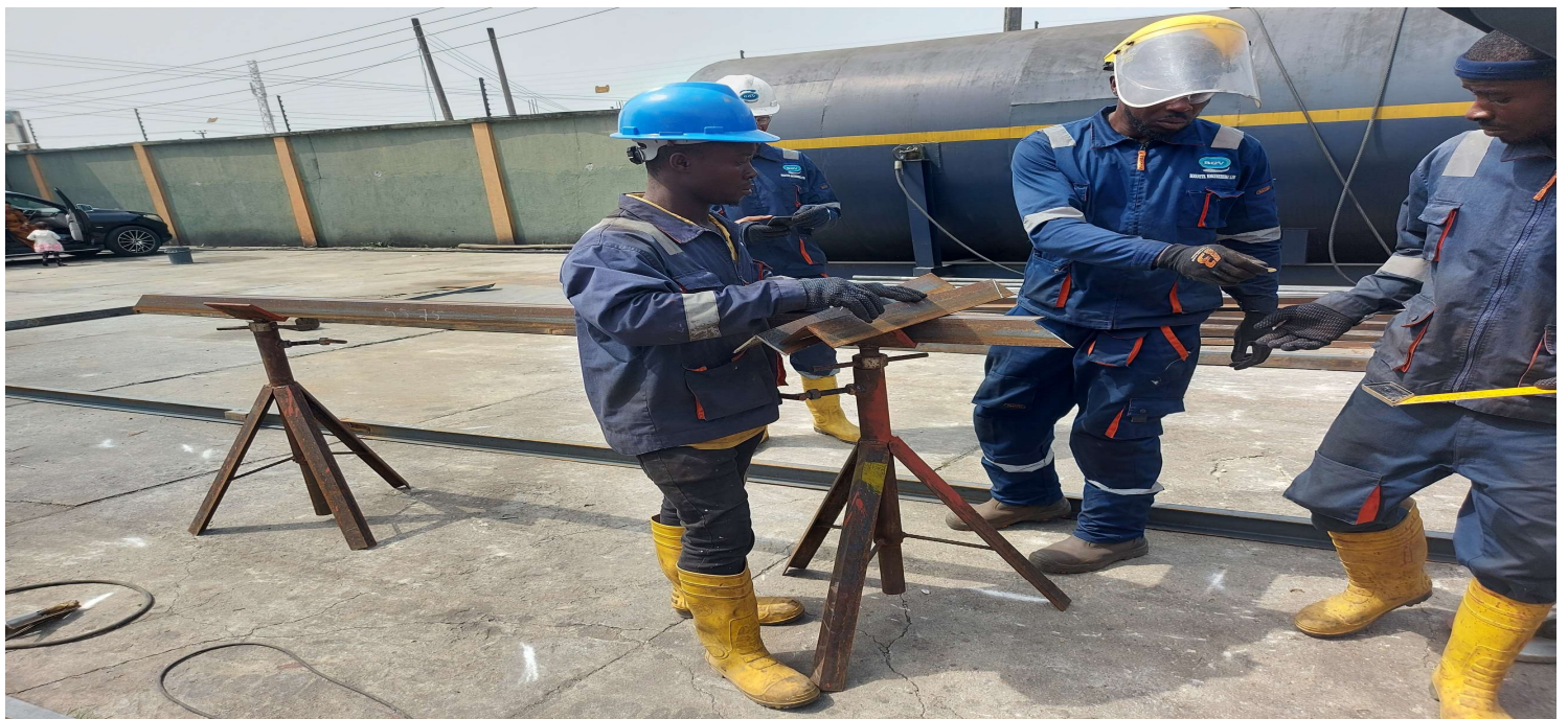
PLATFORM FABRICATION WORK
