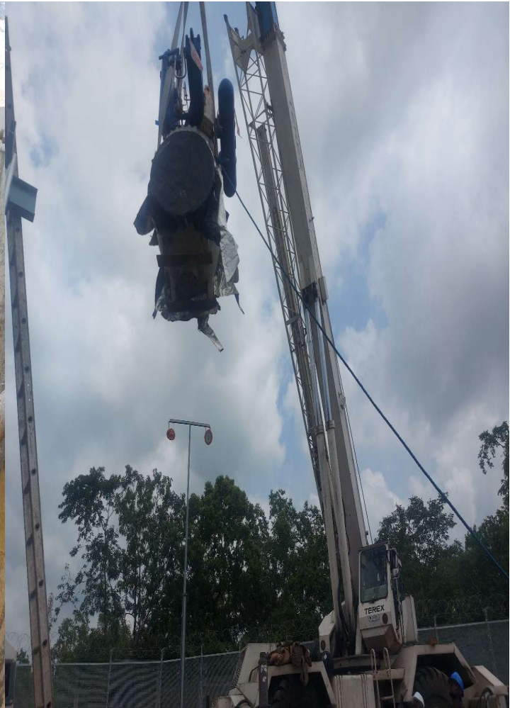
INSTALLATION OF 24 INCHES LINE BREAK VALVE
