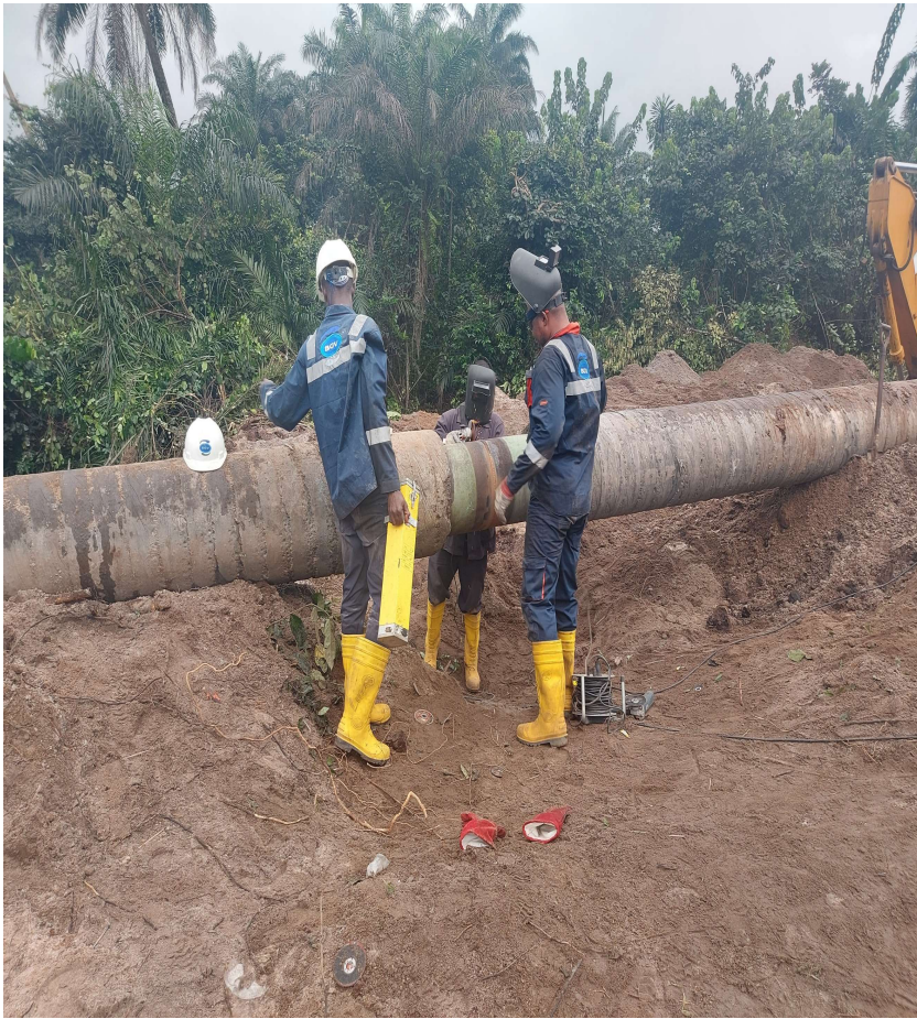
PIPELING RIDGE FORMATION, PIPE LAYING FIT-UP, WELDING, GRINDING
