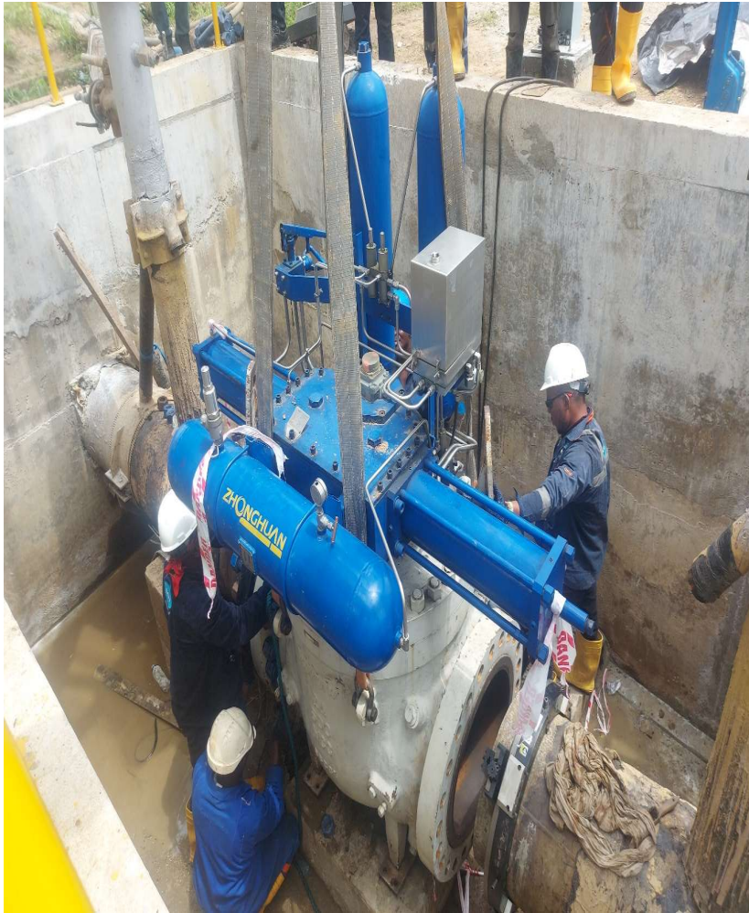
INSTALLATION OF 24 INCHES LINE BREAK VALVE
