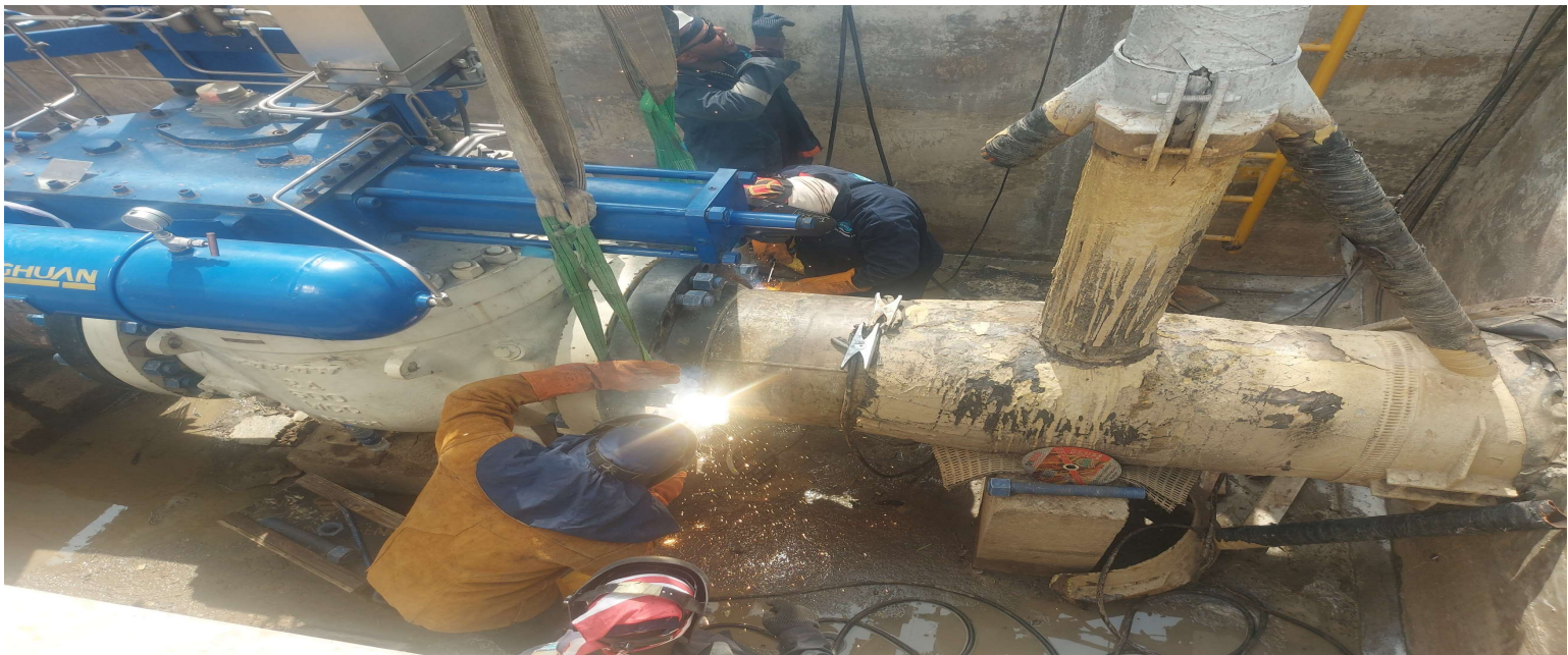
INSTALLATION OF 24 INCHES LINE BREAK VALVE
