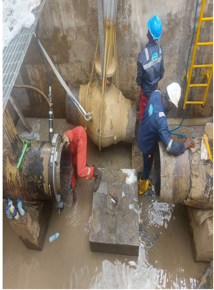
SERVICING OF LINE BREAK VALVE ACTUATOR AND COLD CUTTING OF 24 INCHES WELDONE VALVE
