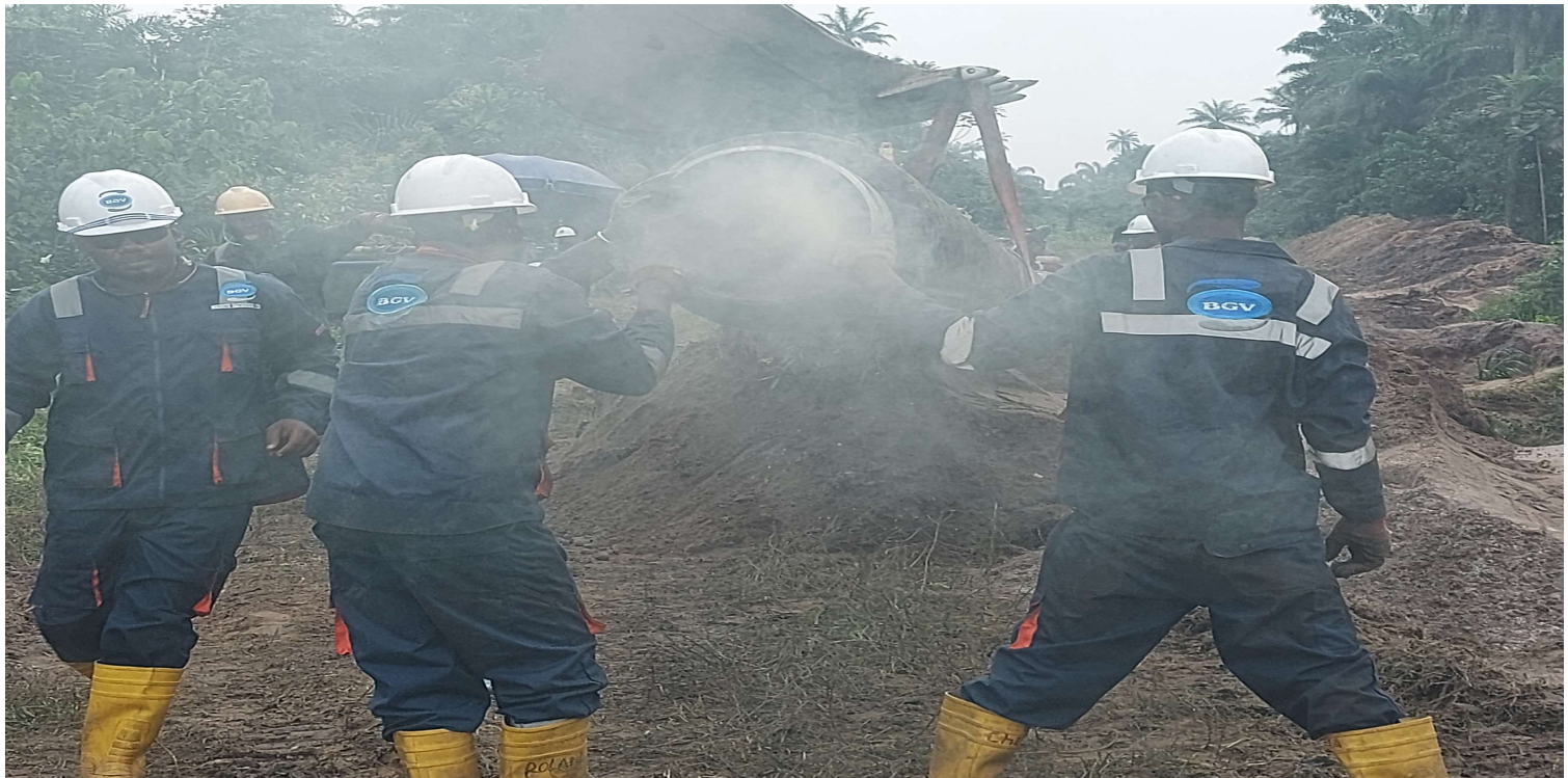
PIPELINE ALIGNMENT AND WELDING DURING PROJECT EXECUTION
