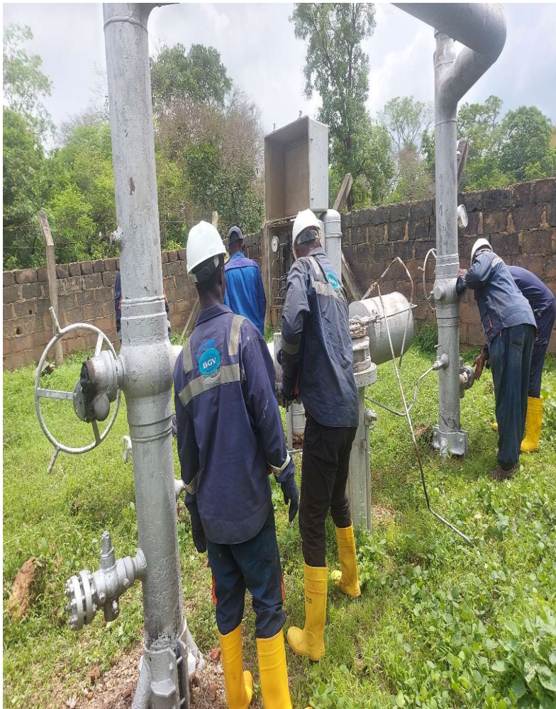
SERVICING OF LINE BREAK VALVE ACTUATOR AND COLD CUTTING OF 24 INCHES WELDONE VALVE
