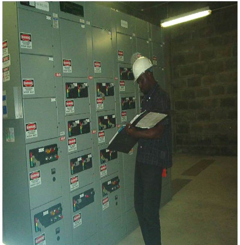
ATCS INSTALLATION PROJECT FOR AGIP
