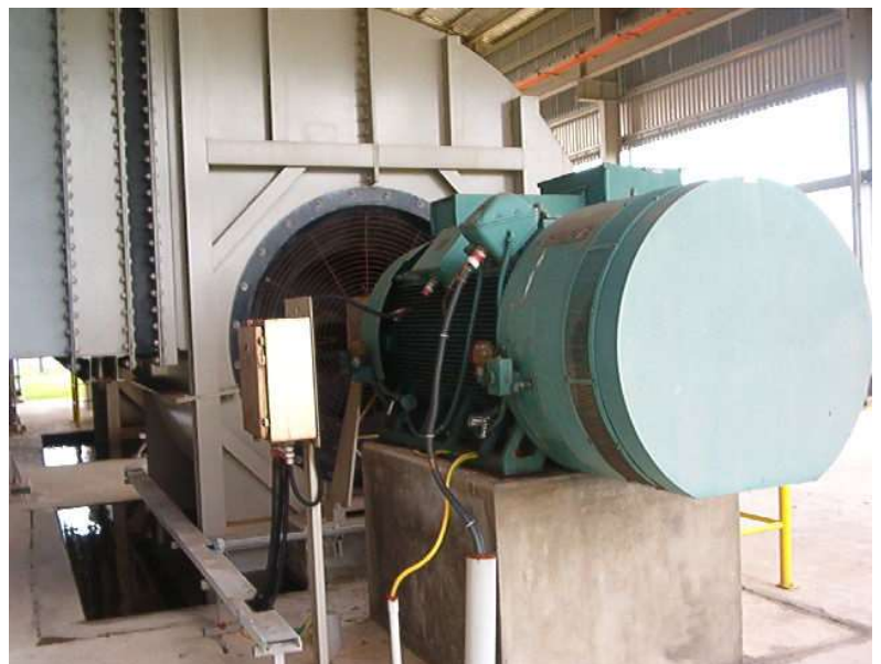
ATCS INSTALLATION PROJECT FOR AGIP
