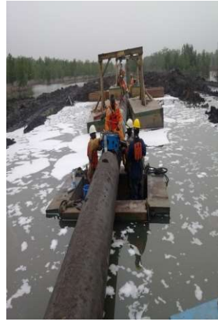
Executed Pipeline Project
