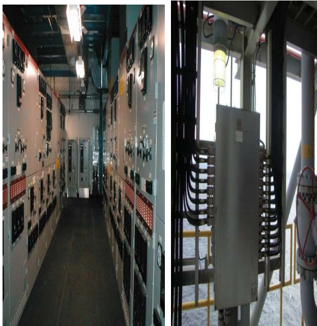
INSTRUMENTATION CABLE INSTALLATION PROJECT FOR GPL
