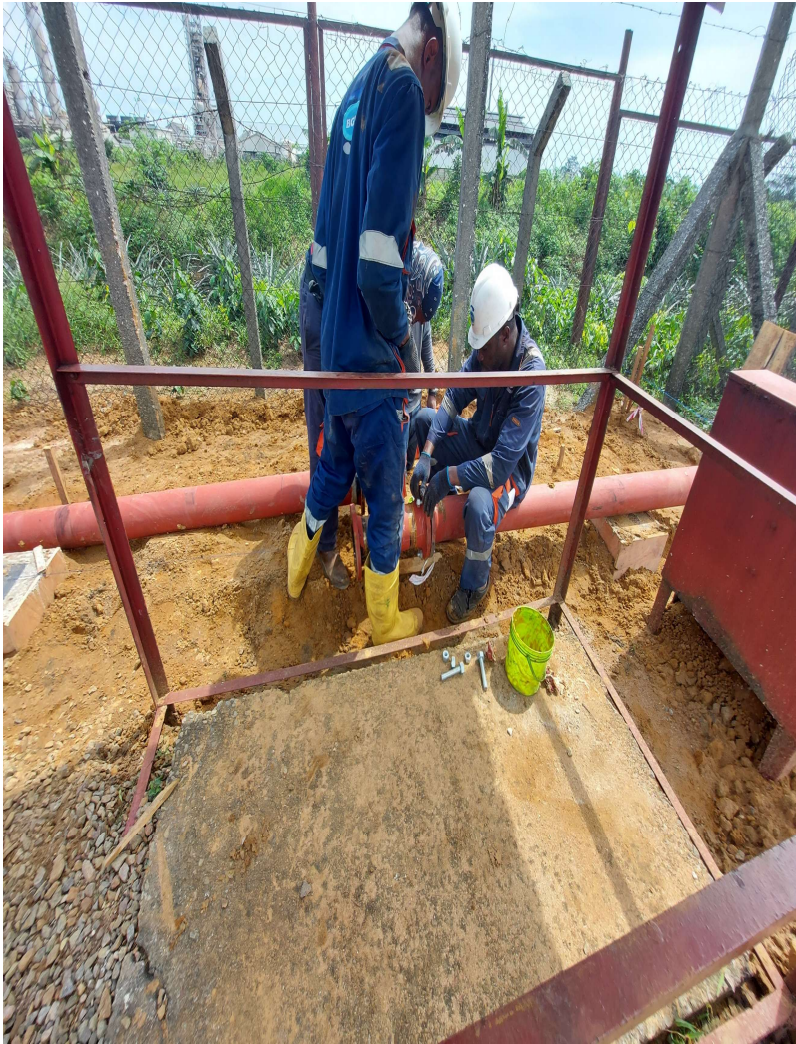
CONSTRUCTION OF ABOVEGROUND FIRE HYDRANT LINE AND RING INSTALLATION
