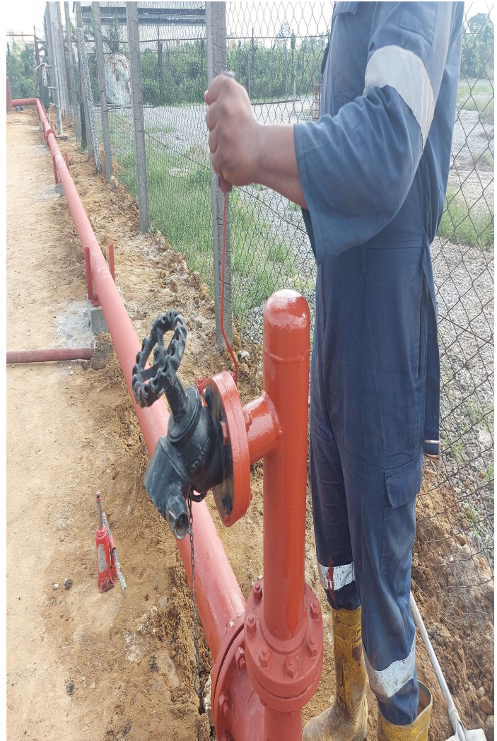
CONSTRUCTION OF ABOVEGROUND FIRE HYDRANT LINE AND RING INSTALLATION
