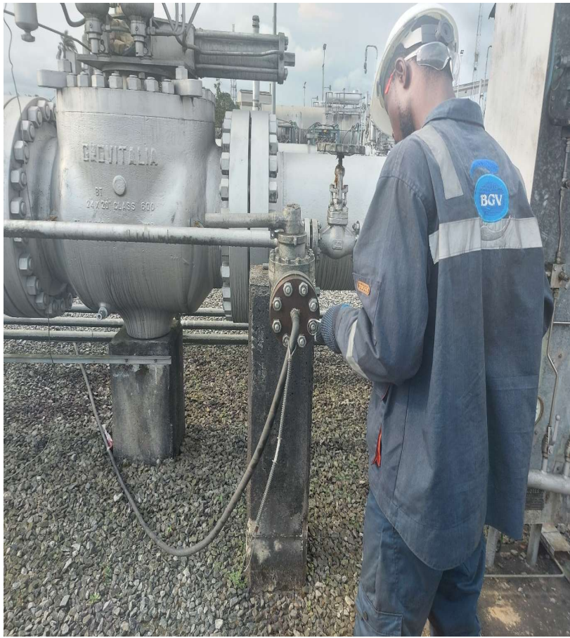
SET-UP OF INJECTION POINT
