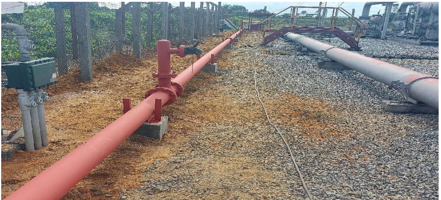
CONSTRUCTION OF ABOVEGROUND FIRE HYDRANT LINE AND RING INSTALLATION
