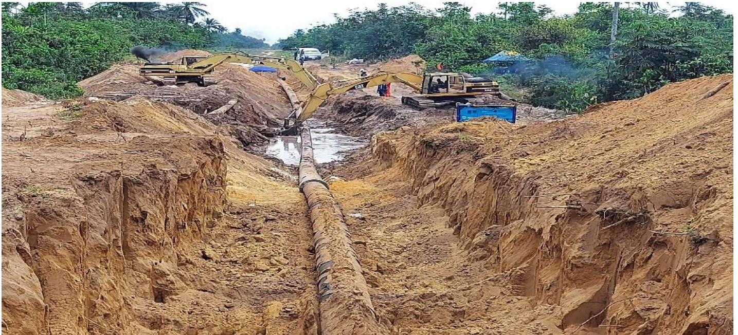
ALIGNMENT OF WELDED LINE PIPES DURING PIPELINE CONSTRUCTION
