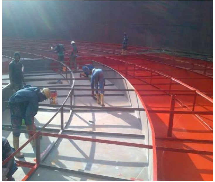
STORAGE TANK 301 – TK – 62 MAINTENANCE PROJECTS
