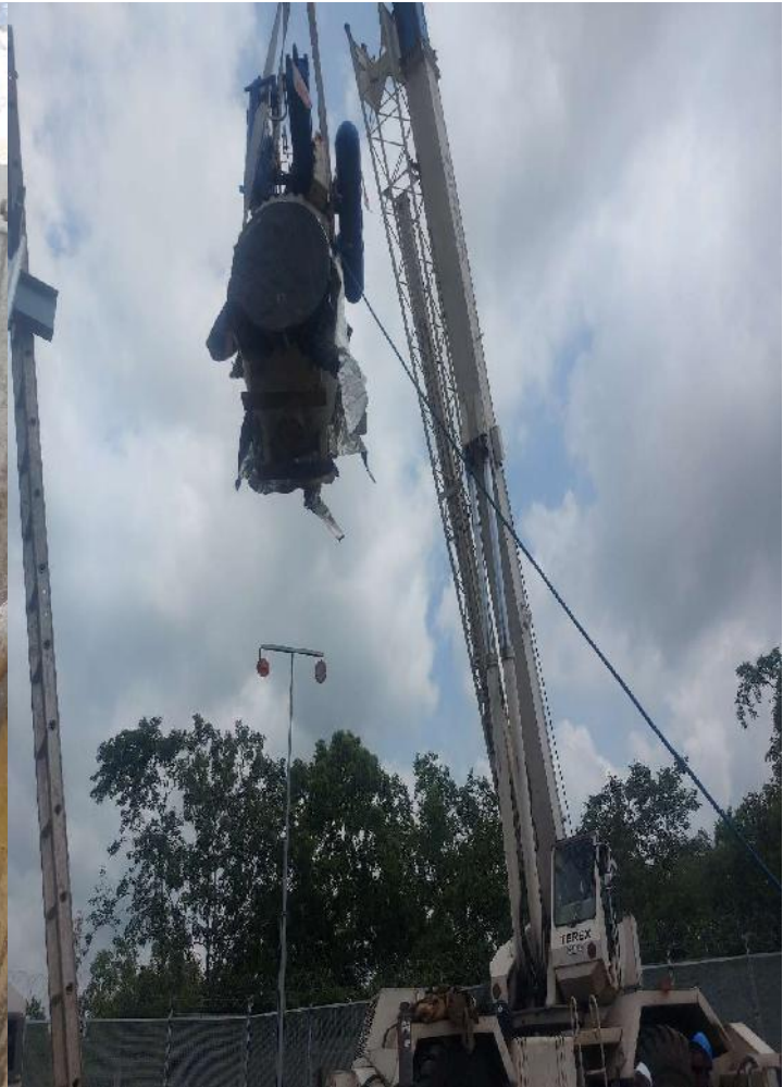
INSTALLATION OF 24 INCHES LINE BREAK VALVE
