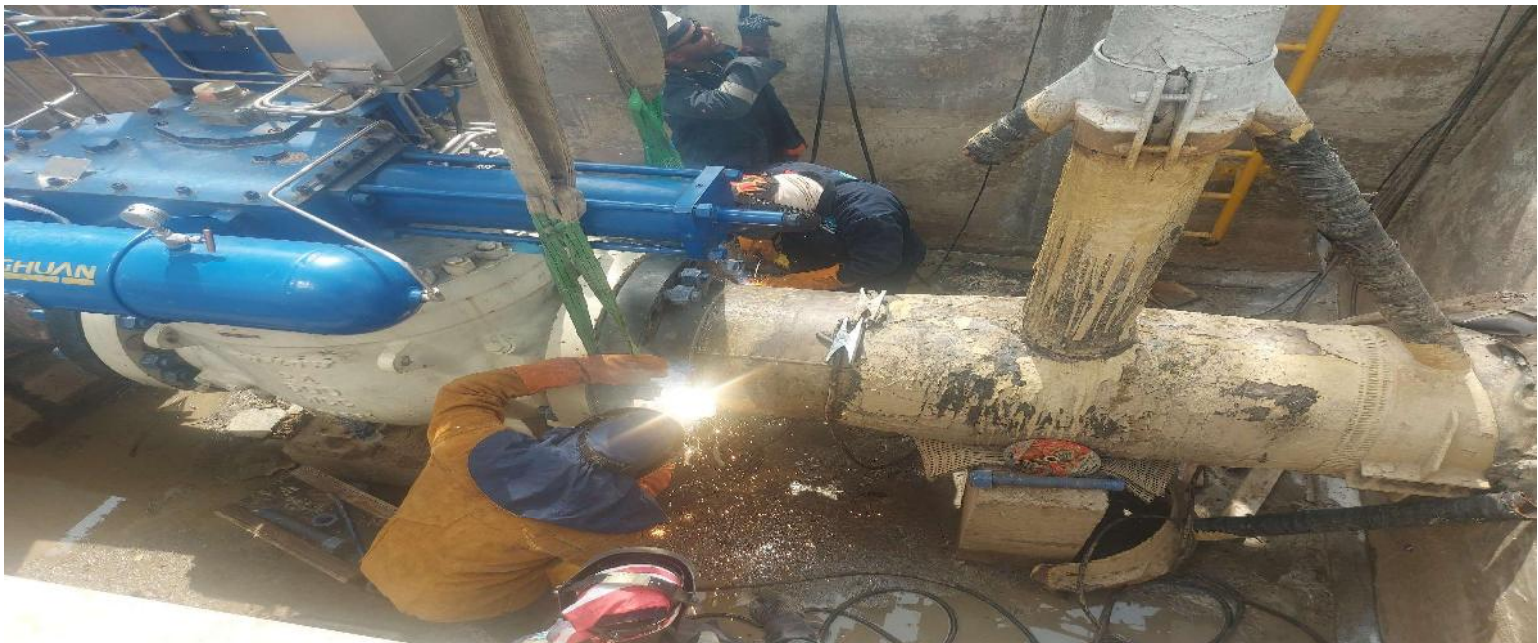
INSTALLATION OF 24 INCHES LINE BREAK VALVE
