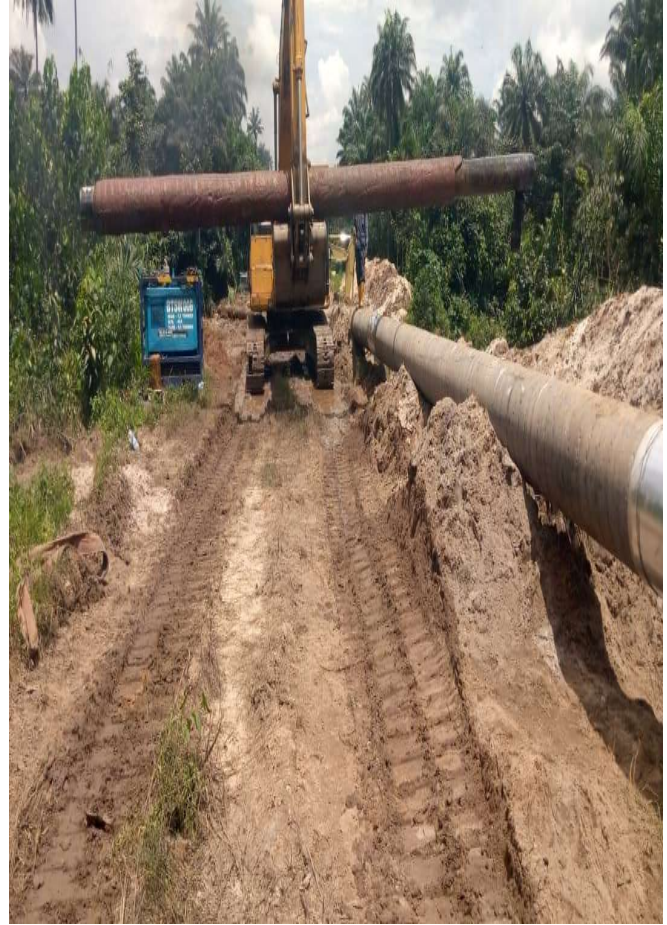
PIPELING RIDGE FORMATION, PIPE LAYING FIT-UP, WELDING, GRINDING
