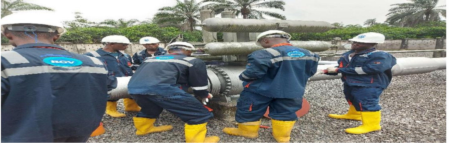
POSITIVE ISOLATION OF PIPELINE BY BLINDING OF ISOLATION VALVE FOR HOT WORK
