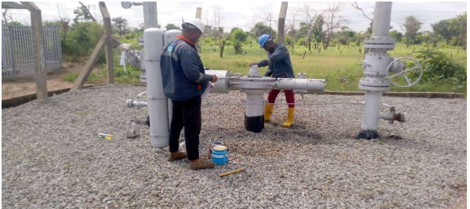
SERVICING OF LINE BREAK VALVE ACTUATOR
