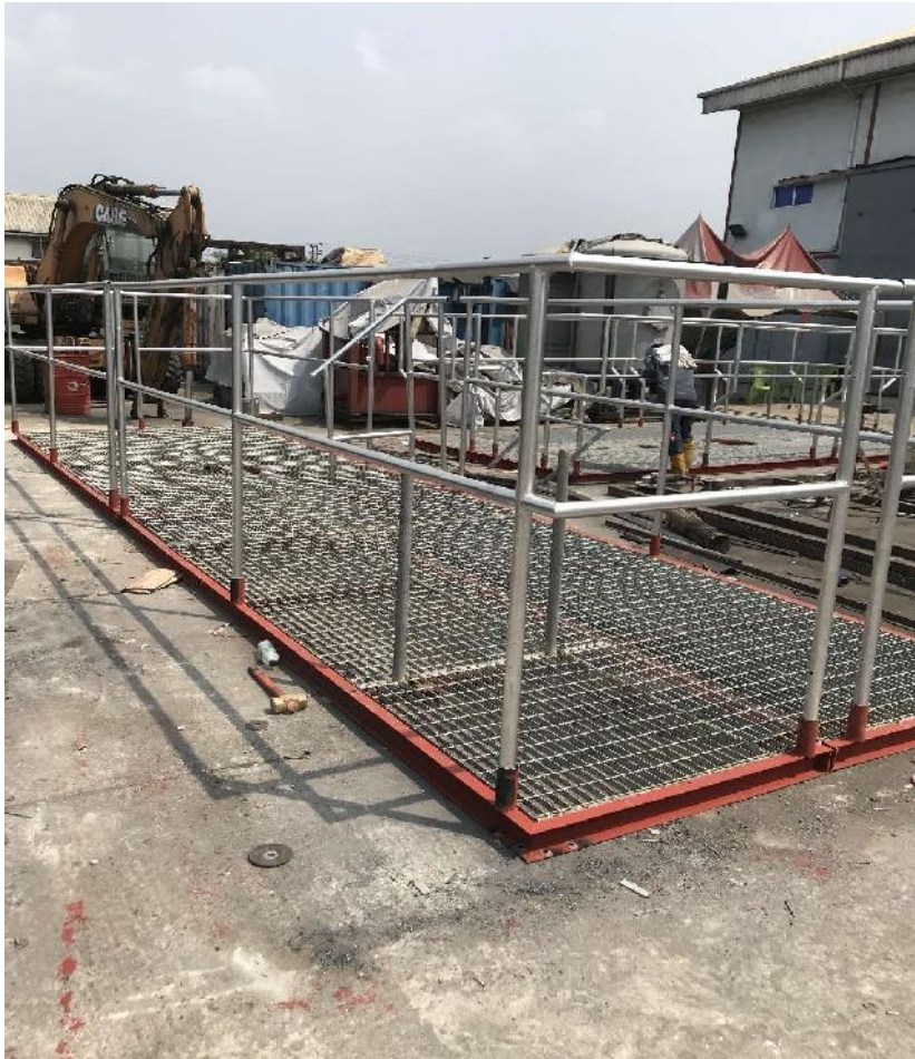
PLATFORM FABRICATION WORK
