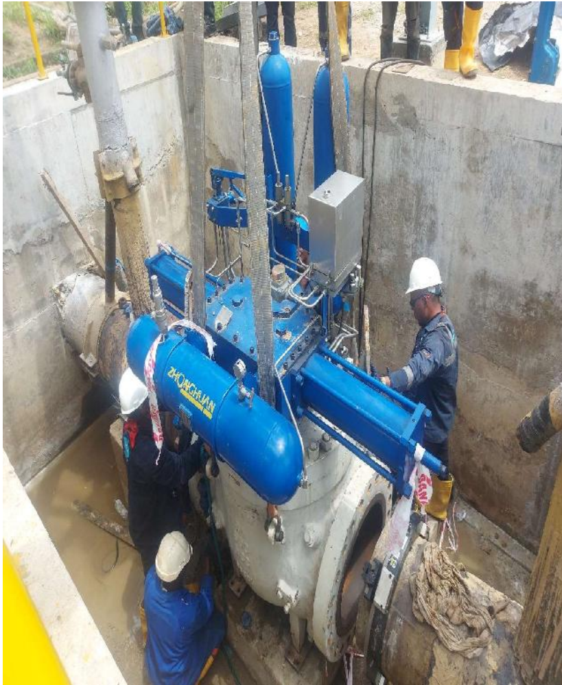
INSTALLATION OF 24 INCHES LINE BREAK VALVE
